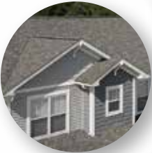
Roofing and Ventilation
