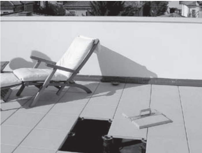
Private terrace - concrete tiles on Eterno pedestals
