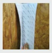
**6.** Remove 3" outside release paper and adhere DuPont™ Flashing Tape to the surface using firm hand pressure or a j-roller – be careful to avoid wrinkles and fish mouths
