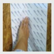
8. Repeat steps 1-7 for the next length of 12" DuPont™ Flashing Tape until reaching the top of the structure. Be sure the 12" DuPont™ Flashing Tape overlaps the previously installed length by a minimum of 2" in a positive shingle fashion.
