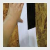
5. Working out from the corner, apply pressure and roll DuPont™ Flashing Tape outward to adhere product smoothly – be careful to avoid wrinkles and fish mouths.
