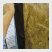
**7.** Remove the remaining 6" release paper and apply the DuPont™ Flashing Tape to the surface using firm hand pressure or a j-roller.
