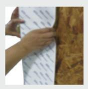
**6.** Remove 3" outside release paper and adhere DuPont™ Flashing Tape to the surface using firm hand pressure or a j-roller. Adhere product smoothly – be careful to avoid wrinkles and fish mouths.
