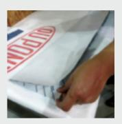
**3.** Starting at the bottom of the wall, place the fold flush against the inside corner with the perforated release papers facing out.
