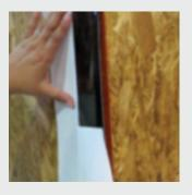
5. Working out from the corner, use firm hand pressure or a j-roller to roll the DuPont™ Flashing Tape outward. Adhere product smoothly – be careful to avoid wrinkles and fish mouths.
