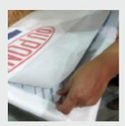
**3.** Starting at the bottom of the wall, align the folded edge with the corner so the perforated release papers are facing out.
