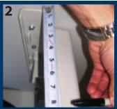
2. Use a marker and mark all four locations to drill. (Image 2) Make sure your hole is a 1/2" below the top lip of the well. This ensures the attachment hardware will be flush with the top lip. (Image 3)
