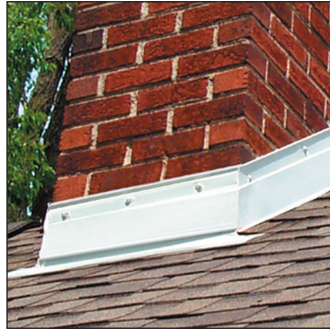
Chimney Flashing
